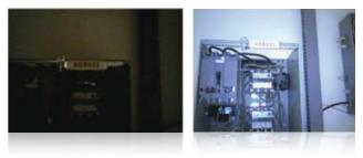
The images are taken with the IR camera's built-in visual camera. The photo on the right is taken with an IR camera that also has LED lights. The visual image on the left is the same target taken with a camera with no LED light. Big difference!
